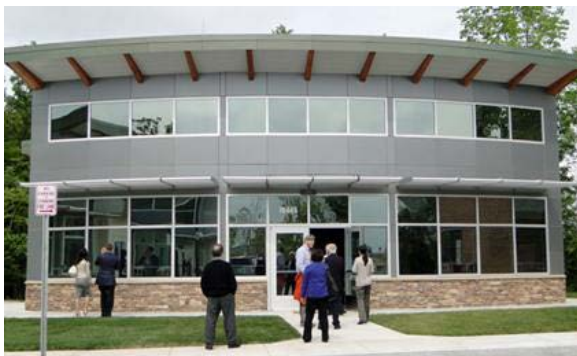
Loudoun County Youth Shelter's new buildings are LEED Gold-rated. (Photo: Lorie Flading, Loudoun County Pub. Aff. & Comm.)
